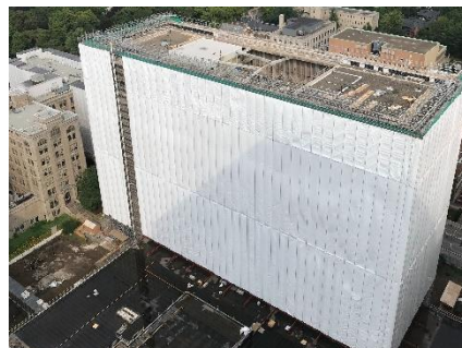
Image: Ferguson Tower envelope scaffolding
